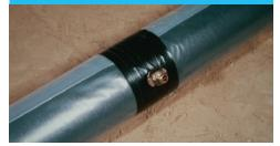
After making the direct service connection, inspect the entire circumferential area for damage and make any necessary repairs.
