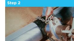
Mount the tapping machine on the pipe area covered by the polyethylene adhesive tape. Then make the tap and install the corporation stop directly through the tape and polyethylene.
