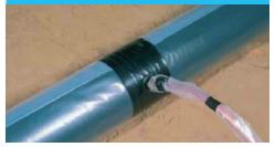
Wrap any connected copper service line within three (3) feet of the pipe with polyethylene.
