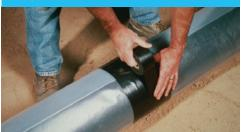
Wrap two or three layers of polyethylene adhesive tape completely around the pipe to cover the area where the tapping machine and chain will be mounted.
