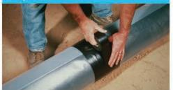
Wrap two or three layers of polyethylene adhesive tape completely around the pipe to cover the area where the tapping machine and chain will be mounted.
