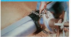
Mount the tapping machine on the pipe area covered by the polyethylene adhesive tape. Then make the tap and install the corporation stop directly through the tape and polyethylene.
