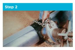
Mount the tapping machine on the pipe area covered by the polyethylene adhesive tape. Then make the tap and install the corporation stop directly through the tape and polyethylene.
