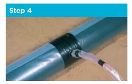
Wrap any connected copper service line within three (3) feet of the pipe with polyethylene.
