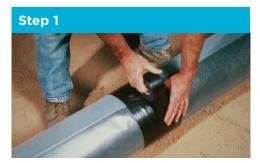
Wrap two or three layers of polyethylene adhesive tape completely around the pipe to cover the area where the tapping machine and chain will be mounted.
