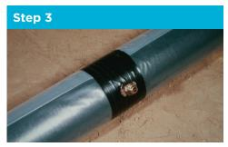
After making the direct service connection, inspect the entire circumferential area for damage and make any necessary repairs.
