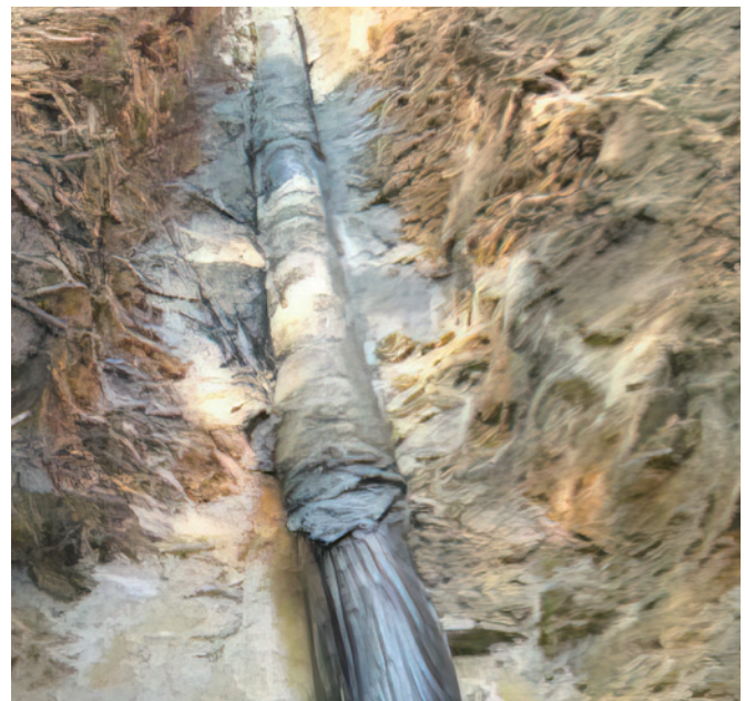
Figure 10: Assembled-line method, pipe built on polyethylene and covered with drilling fluid to facilitate installation
