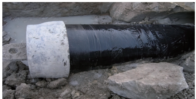
Figure 19: Exposed polyethylene encasement after HDD installation—Polyethylene encasement uncompromised from installation
