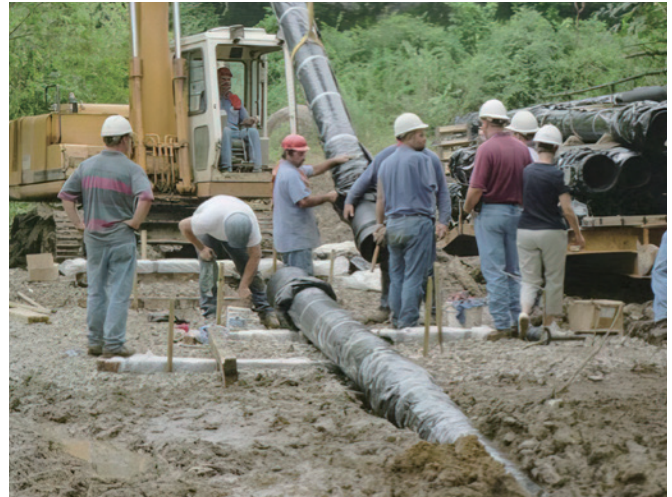
Figure 9: Cartridge method with Ductile iron pipe
