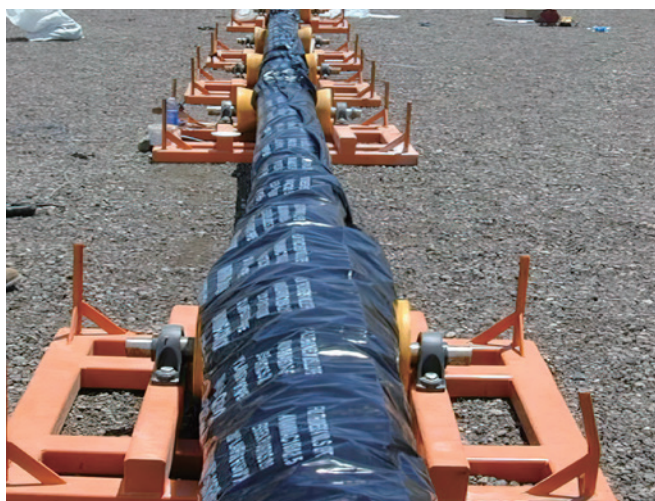
Figure 2: HDD assembled-line method with Ductile iron pipe
