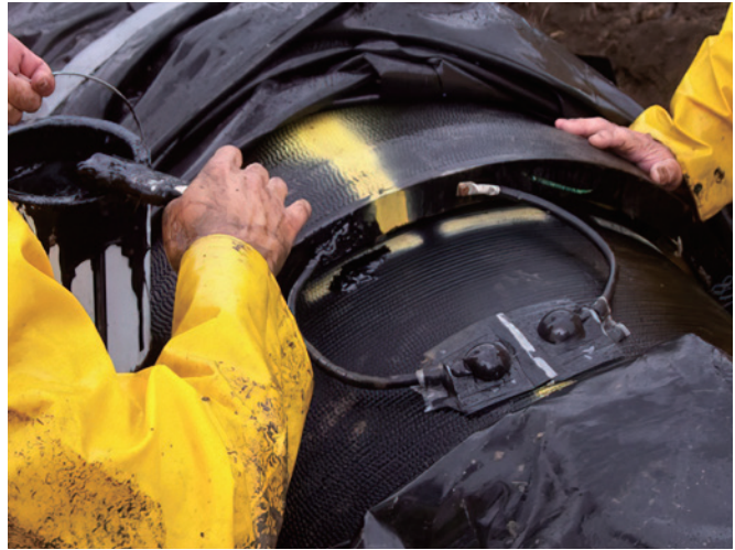
Figure 20: HDD Installation using bonded joints
