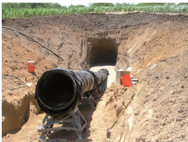
Figure 11: Pipe has been pulled through the bore path, ready to attach to the remainder of the pipeline
