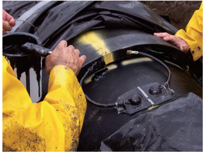
Figure 20: HDD Installation using bonded joints
