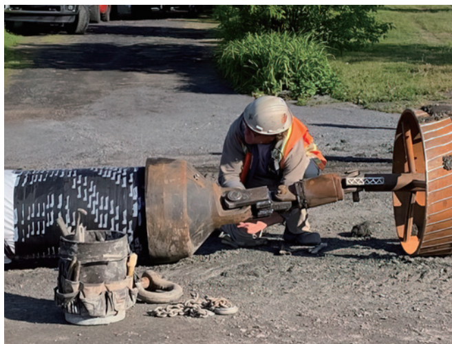
Figure 5: Attaching back reamer and swivel connection to Ductile iron pipe
