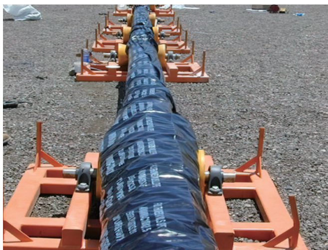
Figure 2: HDD assembled-line method with Ductile iron pipe
