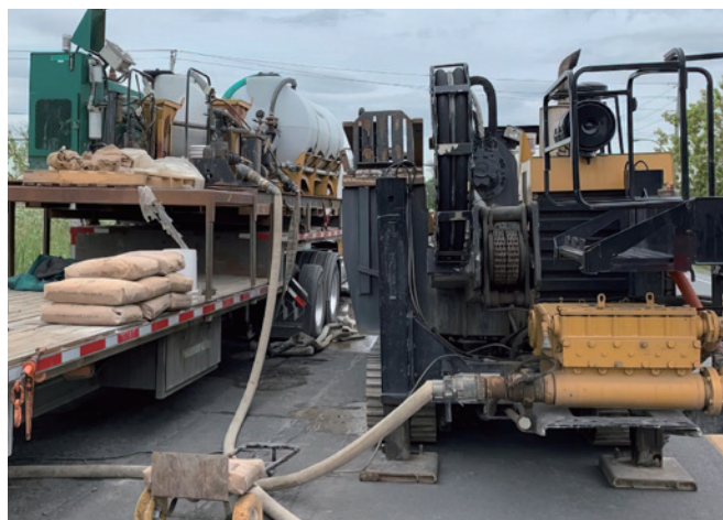
Figure 7: Drilling mud mixing systems
