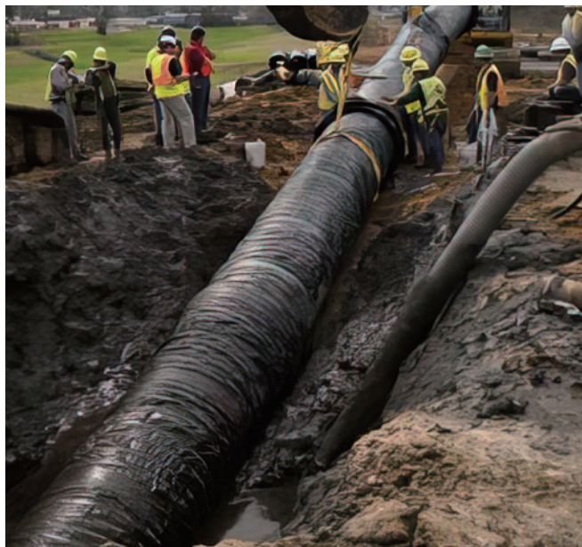
Figure 1: HDD cartridge method with Ductile iron pipe
