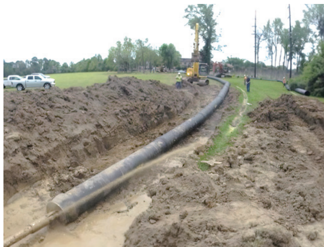
Figure 14: Sweep turns with Ductile iron pipe, shows radius of curvature.
