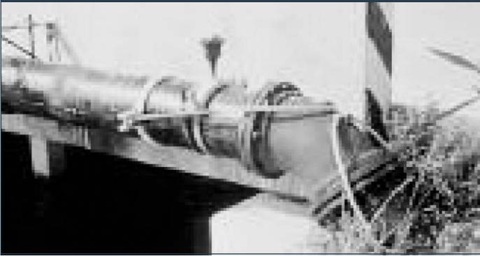
the thrust forces are covered in the DIPRA manual “Thrust Restraint Design for Ductile Iron Pipe.” If desired, a concrete block can be poured to anchor the elbow or bend at the end of the bridge. Sometimes the abutment of the bridge or separate piles can safely be used to “tie-down” the pipeline and/or bends and restrain the thrust forces.
