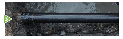
Pipe rewrapped with polyethylene encasement
