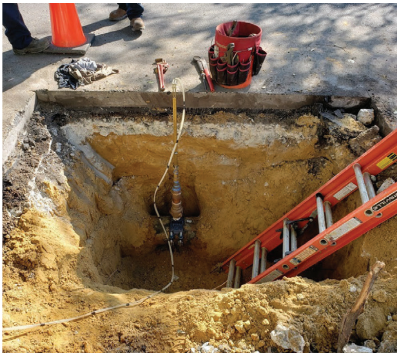
Figure 3: Tapped pipe with pitot rod inserted. Velocity measurements taken at points traversing the inside diameter of the pipe.
