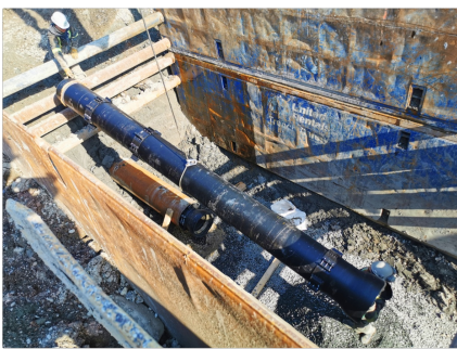
Sliplining Ductile iron pipe inside a steel casing under the road.
