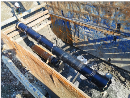
Sliplining Ductile iron pipe inside a steel casing under the road.
