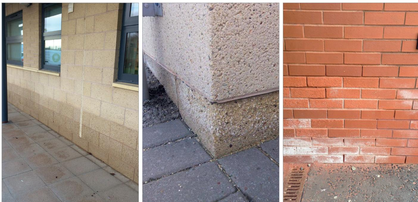
The effect of regular de-icing salts on masonry materials near pavement level.
