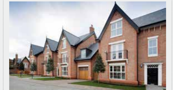
Architect: Calderpeel Architects Brick: Birtley Olde English Buff
