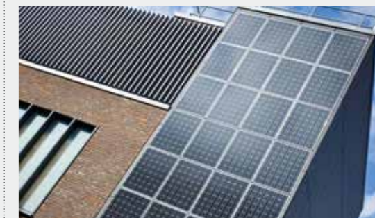
Architect: Marchini Curran Associates Brick: Crowborough Multi Stock
