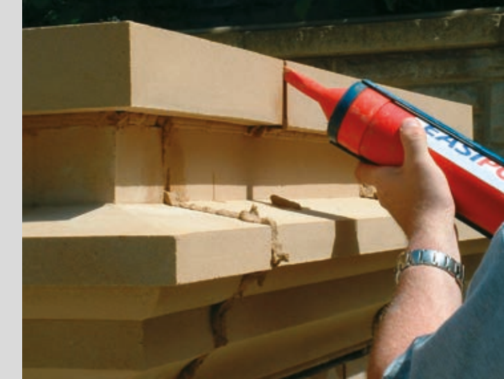
Easipoint mortar during installation.
