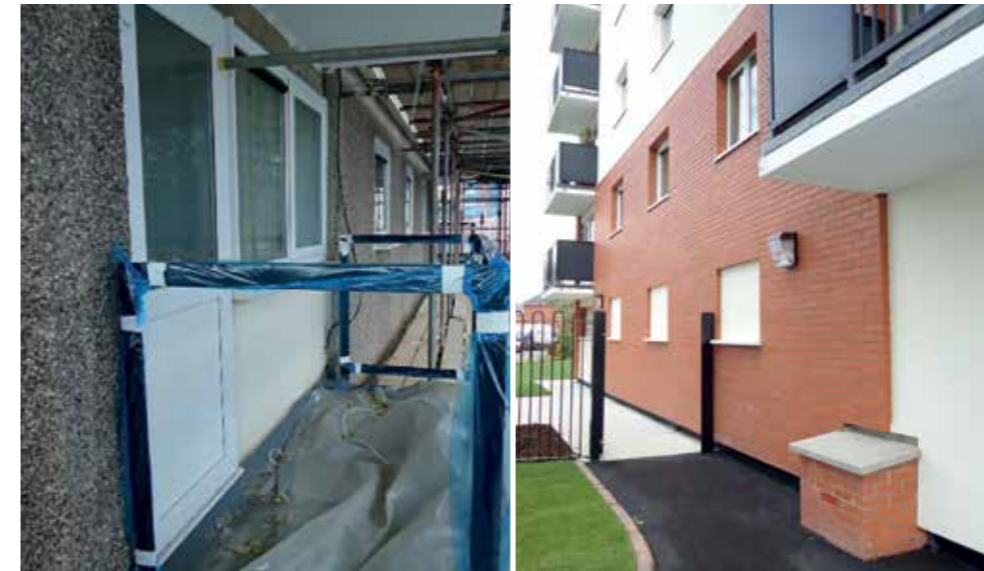
BEFORE REFURBISHMENT OLD NO-FINES FINISH
