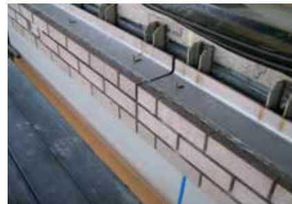
FIXING BRACKET DETAILS
