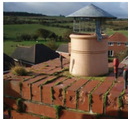
Flat brick on edge is not suitable to cap chimneys. Water is not shed quickly resulting in organic growths and increased likelihood of frost failure.
