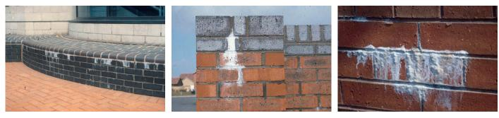
Lime staining is often mistaken as efflorescence, however, it usually emanates from mortar joints and doesn't disappear when wet. Like efflorescence it needs saturation to transport the material, in this case free lime present in mortar or concrete and, as the solution leeches out, it leaves the trailing effect shown above.
