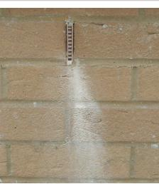
It is often clear where work has been left for the day without covering and a line of lime bleed-out staining appears where a downfall of rain has triggered the process.
