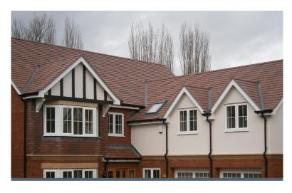
Where a roof design includes details such as hips, valley, or verges, which are positioned close to each other, securing cut tiles can become challenging. Often one or both nail holes, which usually provide a head fixing, require removal during the cutting process.
