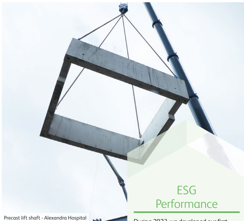
Precast lift shaft - Alexandra Hospital
