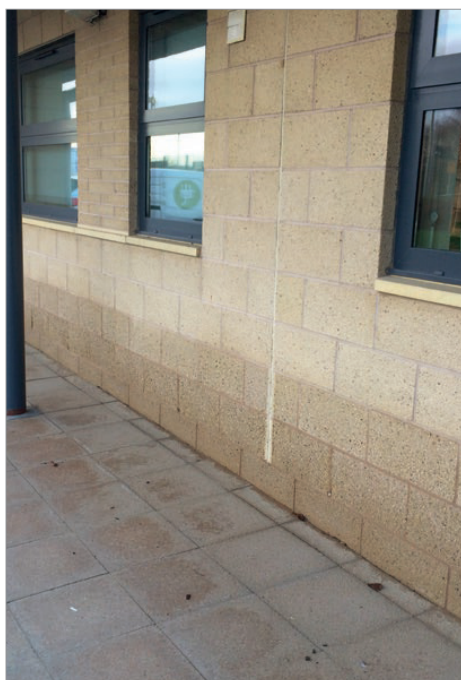
The effect of regular de-icing salts on masonry materials near pavement level.
