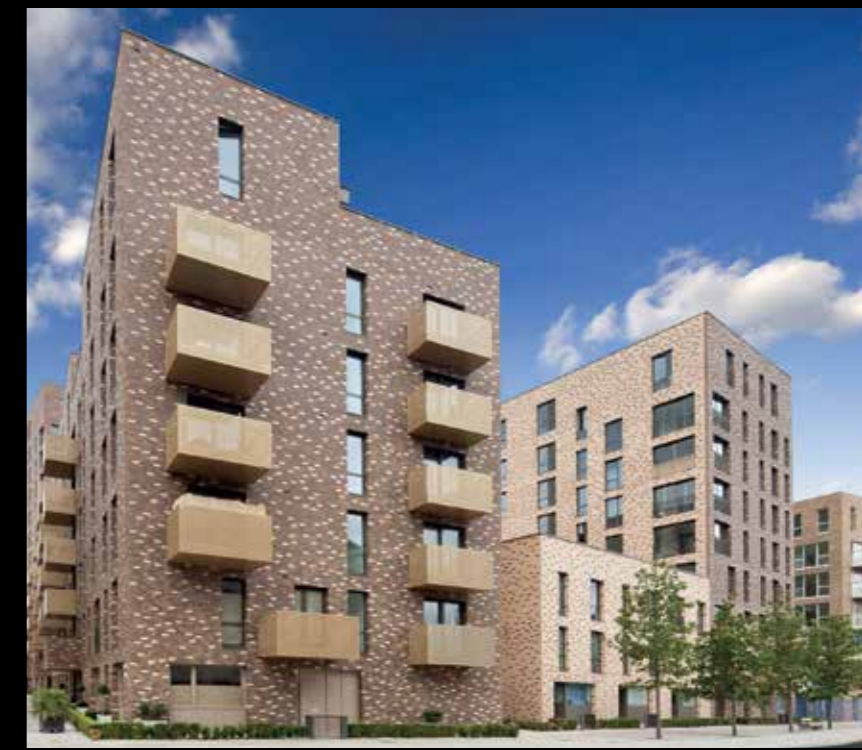
Best Housing Development 26+ Units Union Phase Black B, Devas Street, London E3 | Products: a) Bow Blend: Milburn Ashen Grey Brown, Smooth Buff b) Bromley Blend: Milburn Ashen Grey Brown, Smooth Buff, Cheddar Brown
