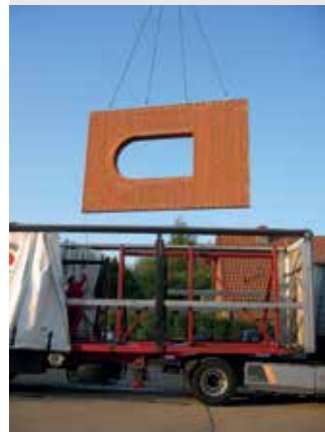
Delivery of panels
