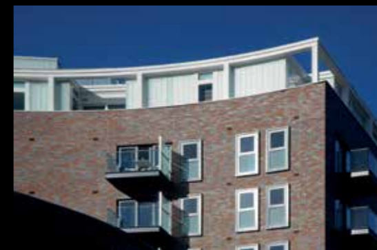
Project 2: Montreal House, Canada Water, Southwark, London SE16 Product: Rotherhithe Blend (Atlas Smooth Red, Staffordshire Smooth, Staffordshire Slate Blue Smooth)
