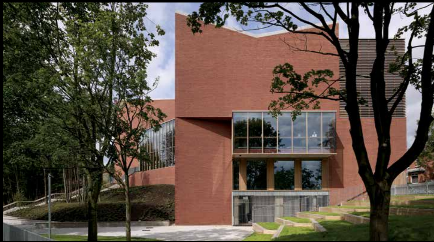
Supreme Winner, Best Public Building & Specialist Brickwork Sub-Contractor (Gilbert Ash NI Ltd) Lyric Theatre, Belfast | Product: Heritage Red Blend
