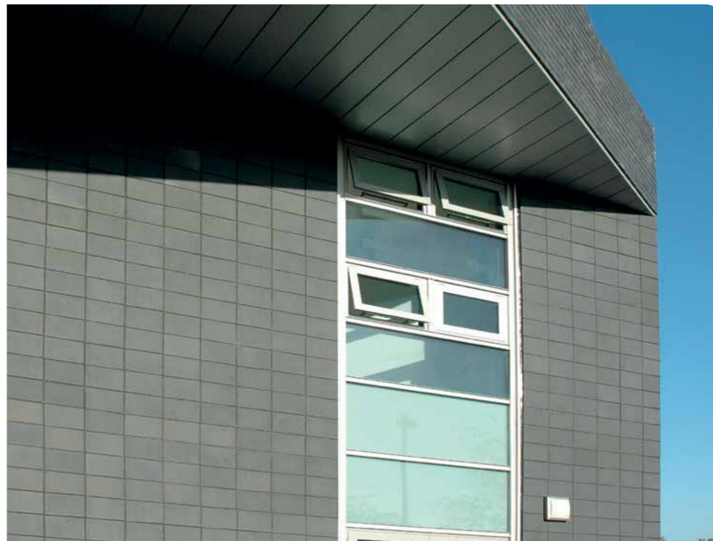
National Trust Headquarters, Swindon | Fireborn® Natural Blue and Staffordshire Slate Blue Smooth
