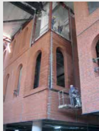
Installation on site
