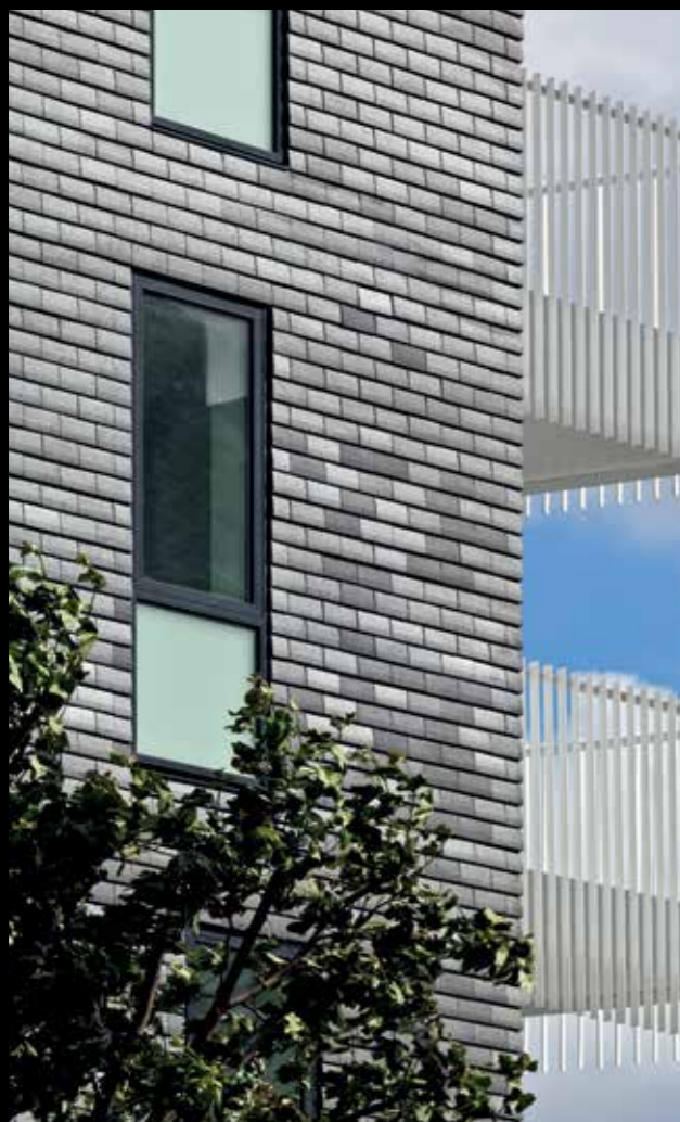
Best Housing Development 6-25 Units Bermondsey Island, Tower Bridge Road, London SE3 Product: Tilebrick™ Smooth Blue
