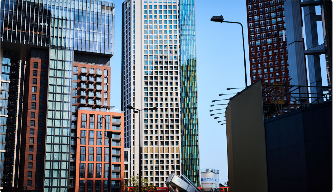
RJ Facade Systems project, Miles Street London scheme comprising of 37 floors of student accommodation using RJ Facades substructure systems to support various facade materials.
