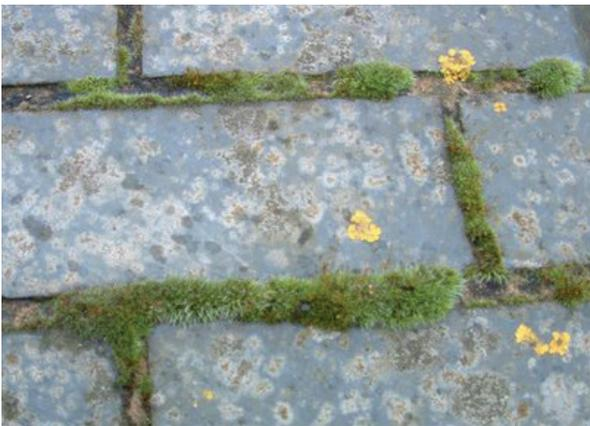
Algae, lichens and mosses are commonly found growing on external surfaces of buildings, particularly where design features or maintenance faults result in frequent wetting of the surface.
