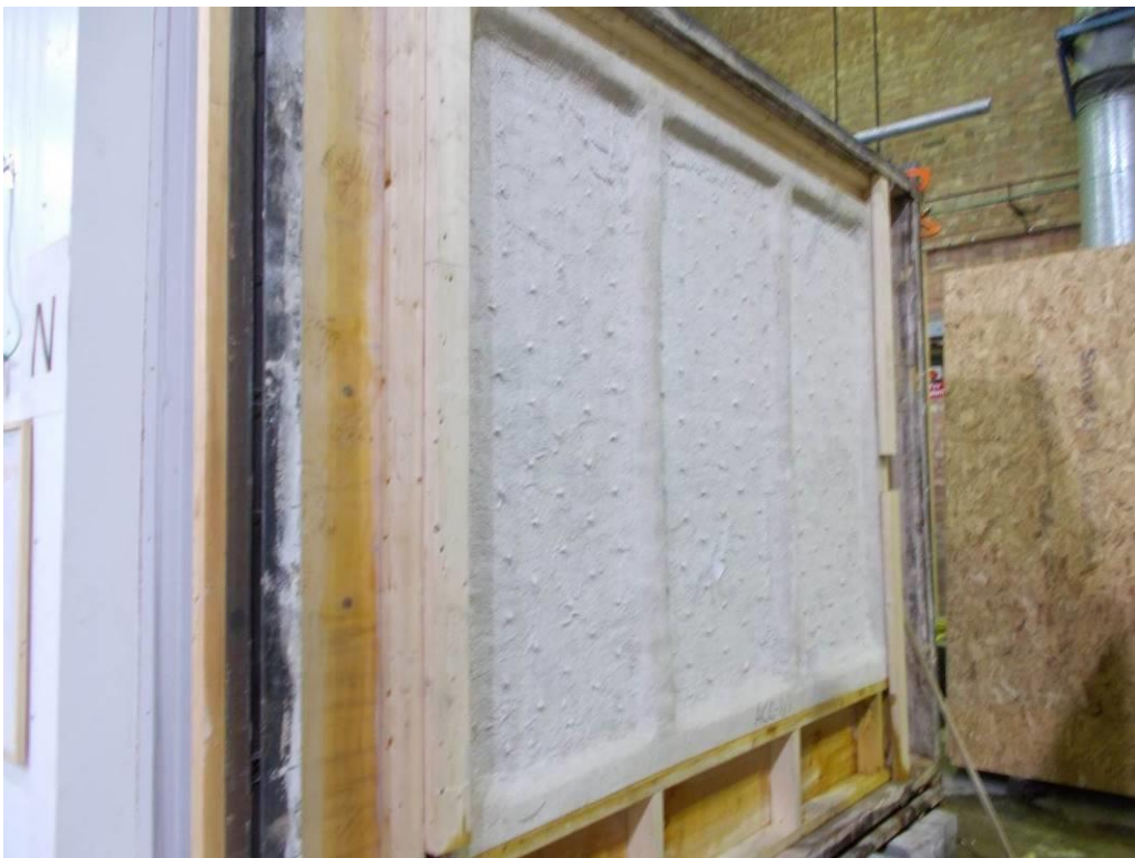
Plate 4 - Rear of Panel Prior to Test
