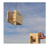
health and safety issues - when compared to traditional construction methods. Our lift shafts are manufactured with a lift pit, door openings, lift cap and lifting beam - all in-factory tested.
