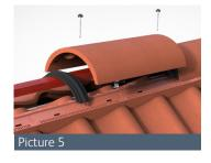
7) Continue fixing nailhole ridge tiles, top fillers and ridge seals along the ridge. If cutting is necessary to maintain the aesthetics of the ridge line, the block end ridge must not be cut. Ridge tiles must not be cut to less than half of their original length. All ridge tiles must be twice fixed with screws supplied (re-drill nailholes if necessary). At the verge, trim the last top fillers and fix the block end ridge tile as described in step 6 to finish the ridge line (Picture 6).
