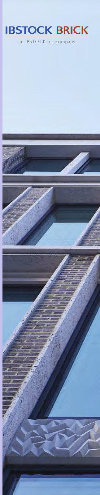
Thirty Broadwick, London, by Emrys Architects (photo: Andy Stagg)
