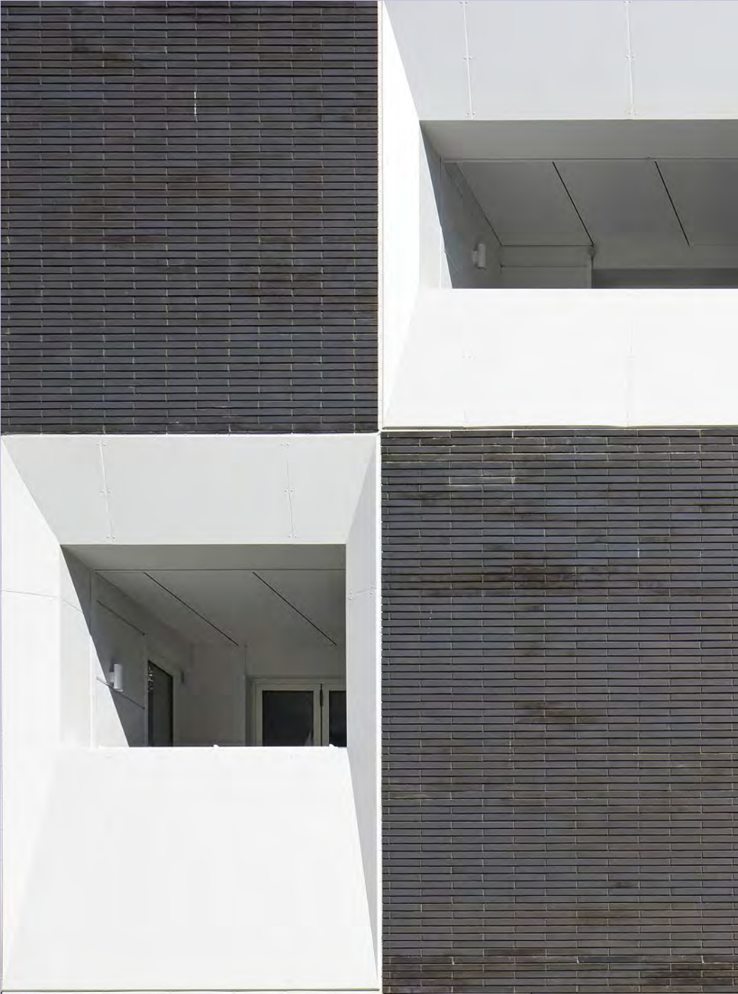
Queen Elizabeth Street, London, by Burwell Deakins (photo: Edmund Sumner)
