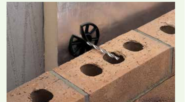
Staifix-Thor TJ2 Helical Wall Tie from Ancon Building Products
