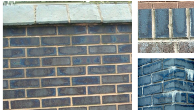
Iridescent appearance caused by light diffraction through fine cementitious material that has leached from mortar
