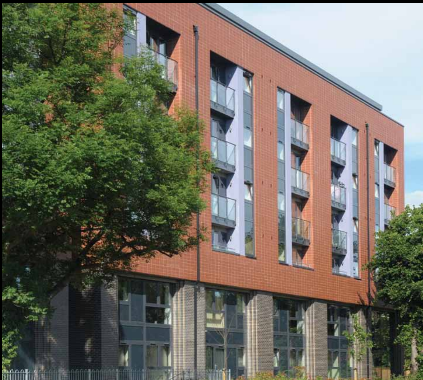
VOLUME HOUSEBUILDER | SENTINEL, WATFORD - FIREBORN NATURAL RED & STAFFORDSHIRE SLATE BLUE SMOOTH
