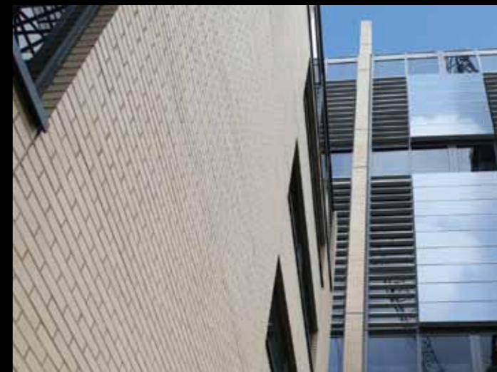
SPECIALIST BRICKWORK CONTRACTOR GRANGE TOWER HOTEL - SMOOTH BUFF
