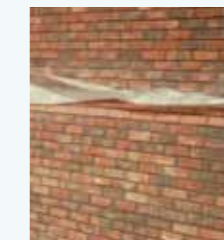
Polythene sheeting minimises staining from work carried out higher up.
