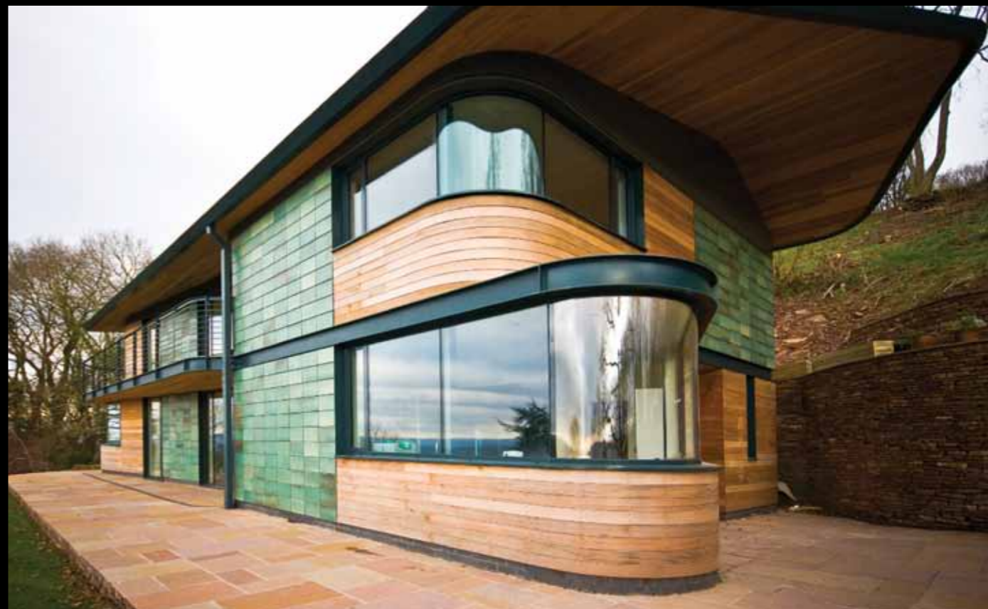
INNOVATIVE USE OF BRICK | BLUE DOOR - ELEMENTIX COPPER
