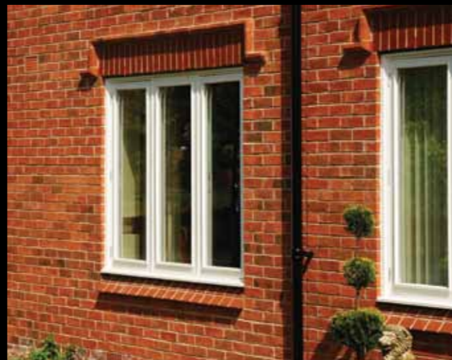
HOUSING 6 - 25 UNITS WATER STREET, PORT SUNLIGHT - COMMERCIAL RED & ATLAS SMOOTH RED
