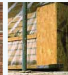
Plywood sheeting protects vulnerable brickwork from knocks.
