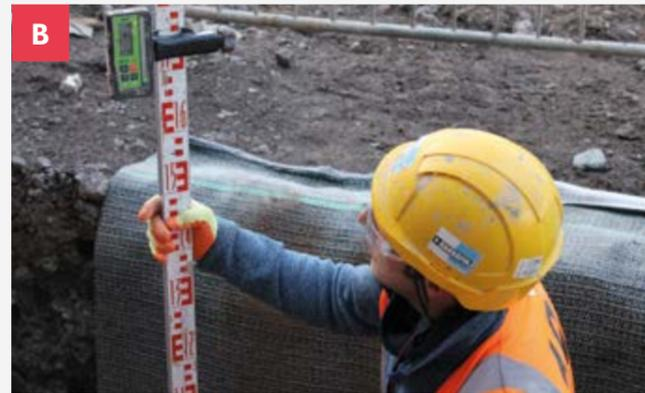
2. Position trough using cast in lifting sockets to required line and level.
