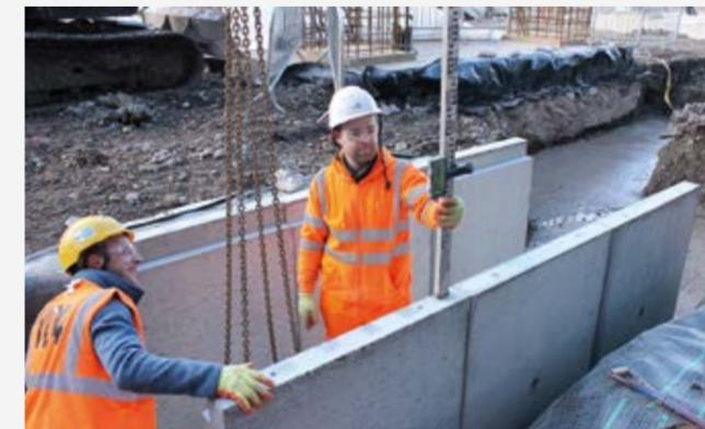
6. Carefully place suitable backfill material around trough to re-form required finished levels.
