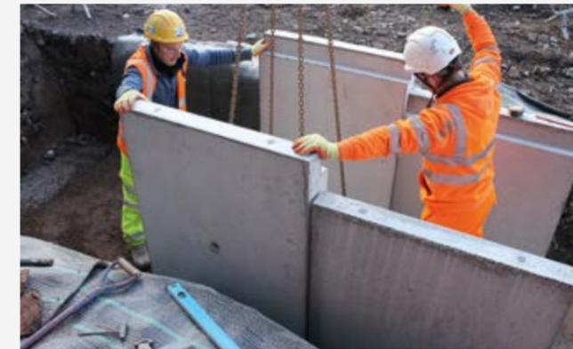
4. Place stone/concrete haunching to sides of trough as installation proceeds and where required.
