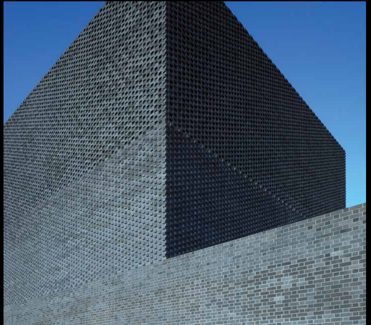
OLYMPIC VILLAGE SUBSTATION, STRATFORD, LONDON | HIMLEY EBONY BLACK
