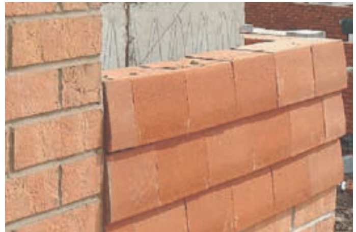
Protect brickwork from the elements
