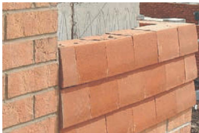
Protect brickwork from the elements
