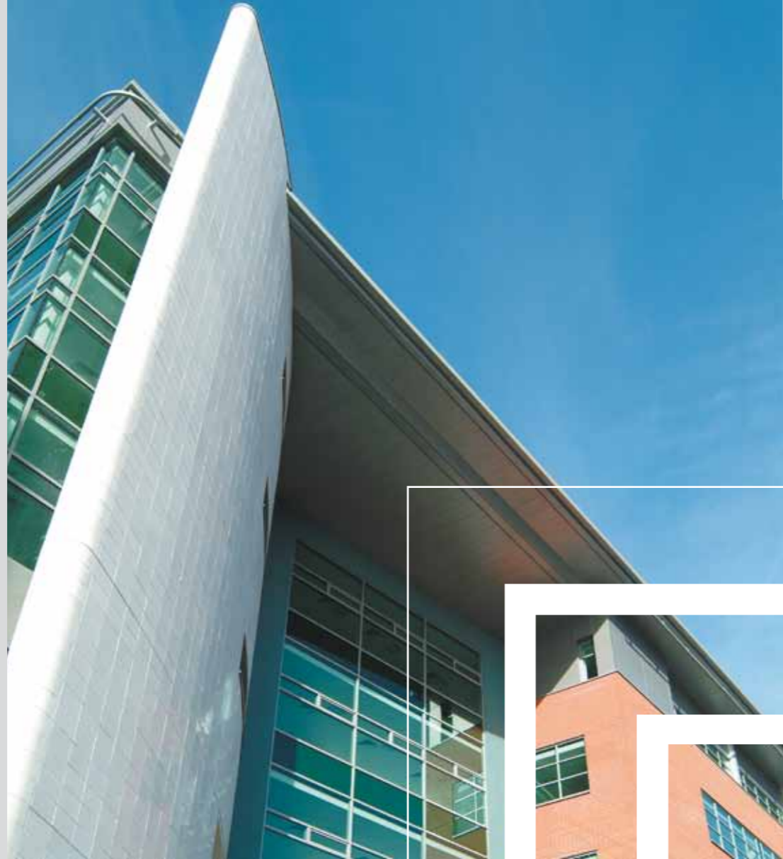
Medici masonry, Twelve Princess Dock, Liverpool
