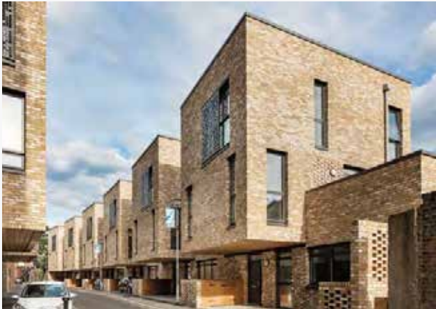
Creek Road, Architect's Choice Award winner at the Brick Awards 2018, utilised Ibstock Funton Old Chelsea Yellow brick to mirror the existing bricks whilst adding a contemporary twist.
