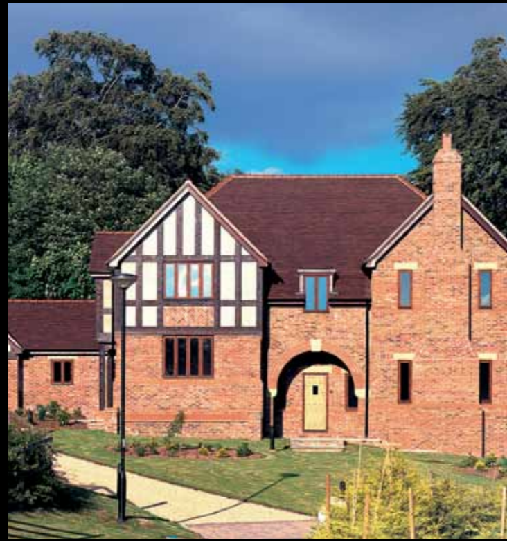
CHAILEY STOCK | PRIVATE HOUSING, HULL, EAST YORKSHIRE
