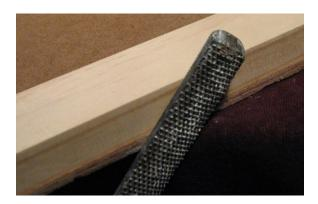
Clean up edges and corners with a file or sandpaper so all joints are flush. Prime panel as desired.
