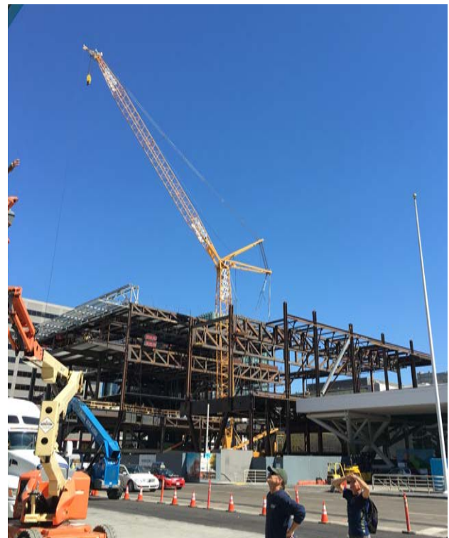
Exterior construction on the Moscone Center
