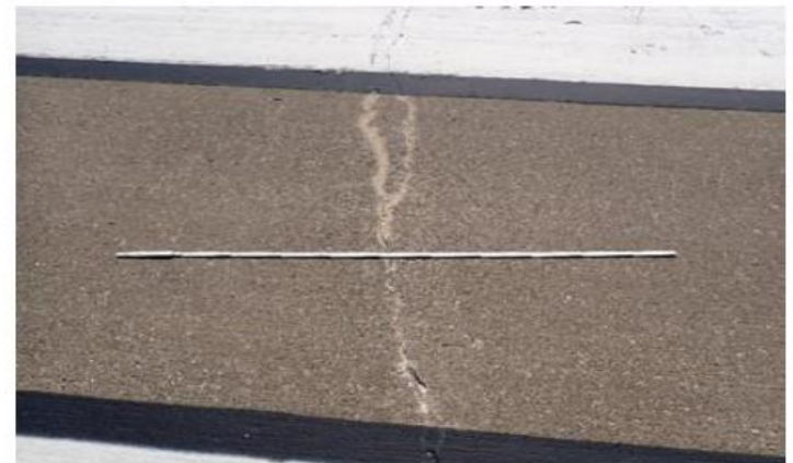
Figure 4-5: CRCP linear cracking on RW 4-22
