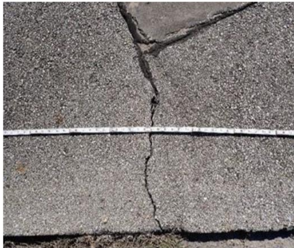
Figure 4-1: Linear cracking, southernmost 1,000' of runway shoulder
