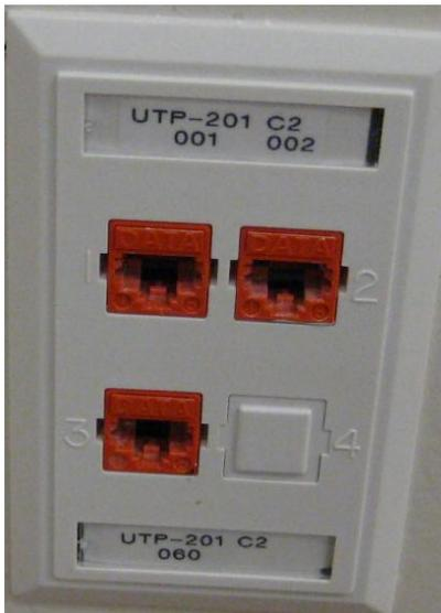
4. Outlet label placement 6-port: under top-aligned, Plexiglas cover – servicing IDF identifier over port identifiers. Ports should be identified left-to-right. Any mid-faceplate ports will require an adhesive label - servicing IDF identifier over port identifiers. Ports should be identified left-to-right. Under bottom-aligned, Plexiglas cover – servicing IDF identifier over port identifiers. Ports
