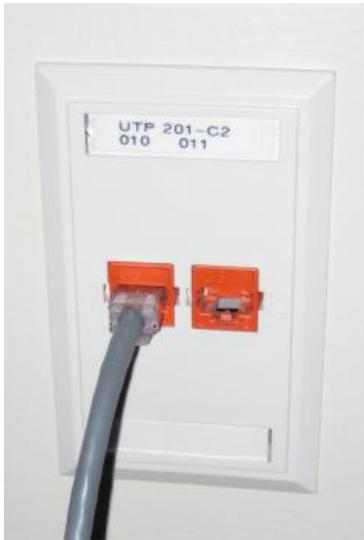
2. Outlet label placement 3-port: under top-aligned, Plexiglas cover – servicing IDF identifier over port identifiers. Ports should be identified left-to-right. Under bottom-aligned, Plexiglas cover – servicing IDF identifier over port identifiers. Ports should be identified left-to-right.
