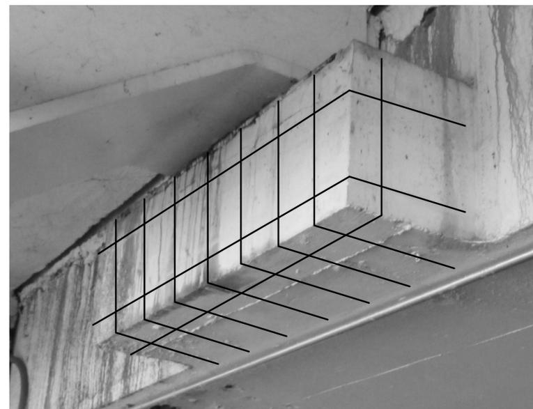
**7** EXISTING CORBEL - REBAR IDENTIFIED DURING GPR TESTING (Approximate Locations)
