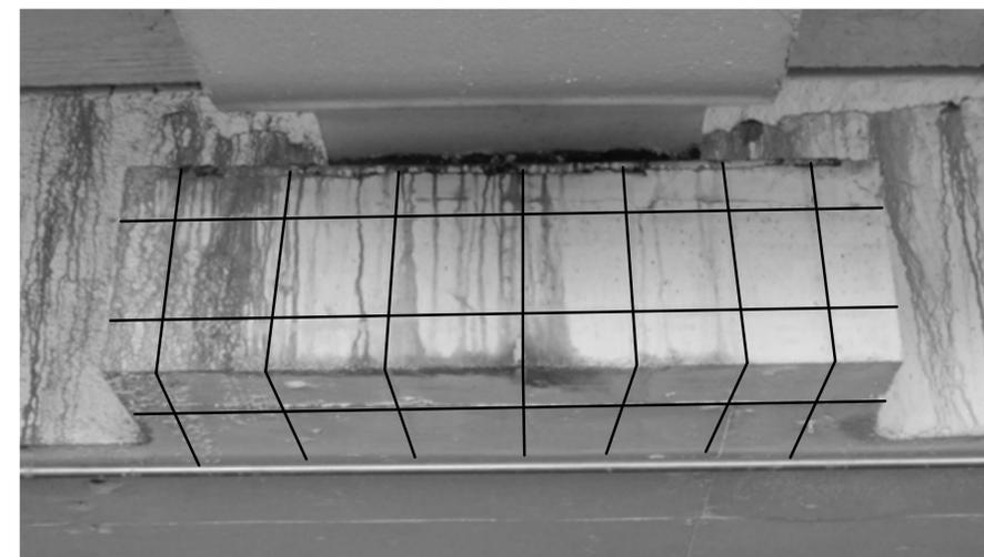
**11** EXISTING CORBEL - REBAR IDENTIFIED DURING GPR TESTING (Approximate Locations)
