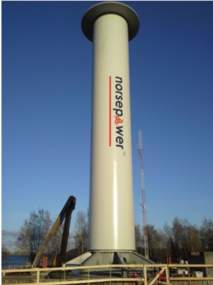
The Norsepower test site in Naantali, Finland
