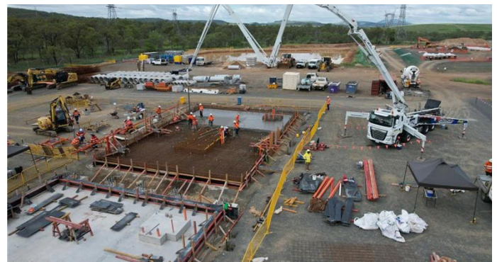
Stanwell's coal combustion products (CCPs) find new life in one of the concrete slabs for the Stanwell Battery laydown area.
