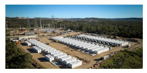
The Tarong BESS is a 300MW / 600 MWh (two-hour duration) lithium-ion battery that is under construction within the Tarong Power Station precinct.
