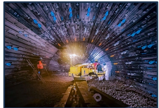
Composite liners installed in operation
