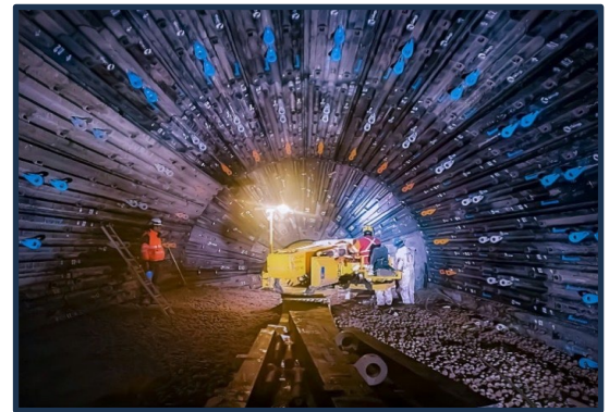
Composite liners installed in operation
