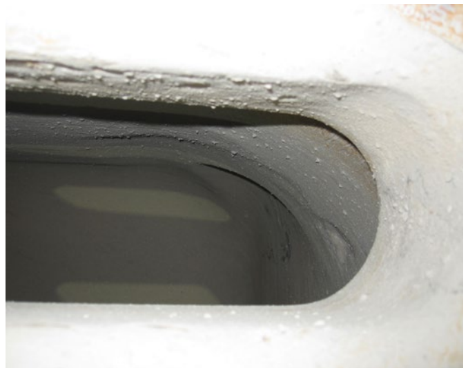
Figure 7 – High Concentrated Wear in the Discharge End Outer Pulp Lifter
