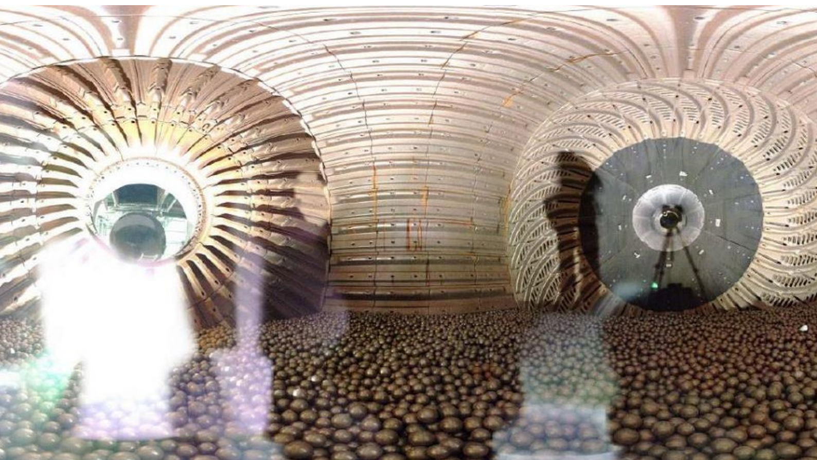
Figure 19 – The New Stage 1 Liner Designed Installed in April 2018
