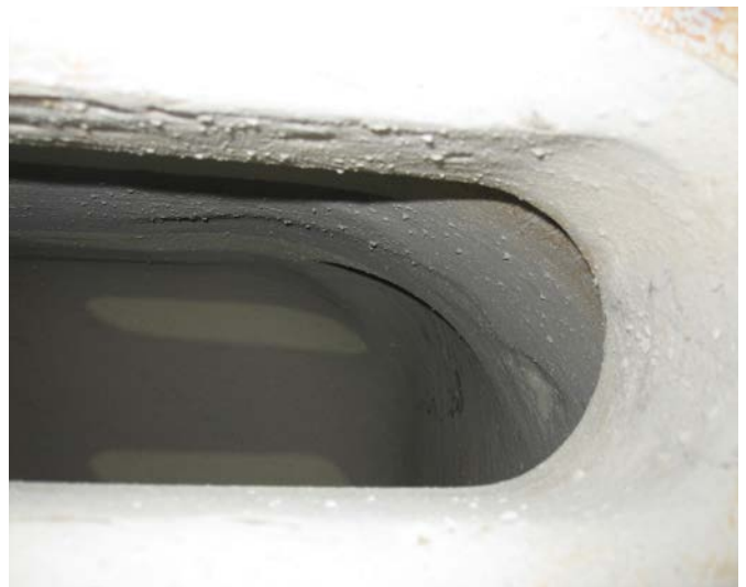
Image 5 – High Concentrated Wear in the Discharge End Outer Pulp Lifter
