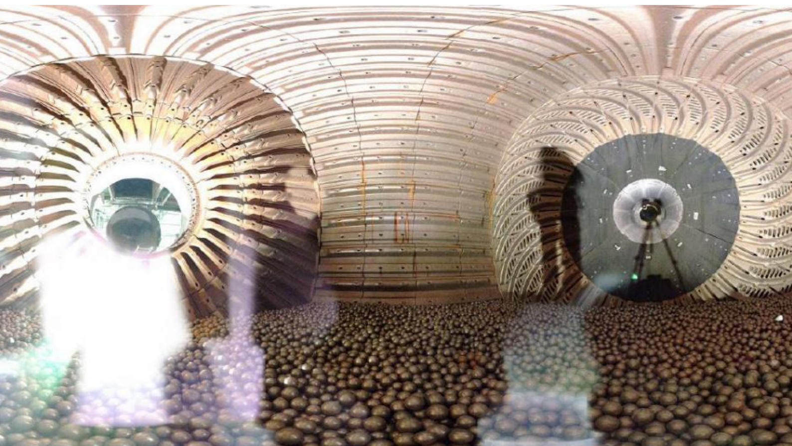
Image 7 – The New Stage 1 Liner Designed Installed in April 2018
