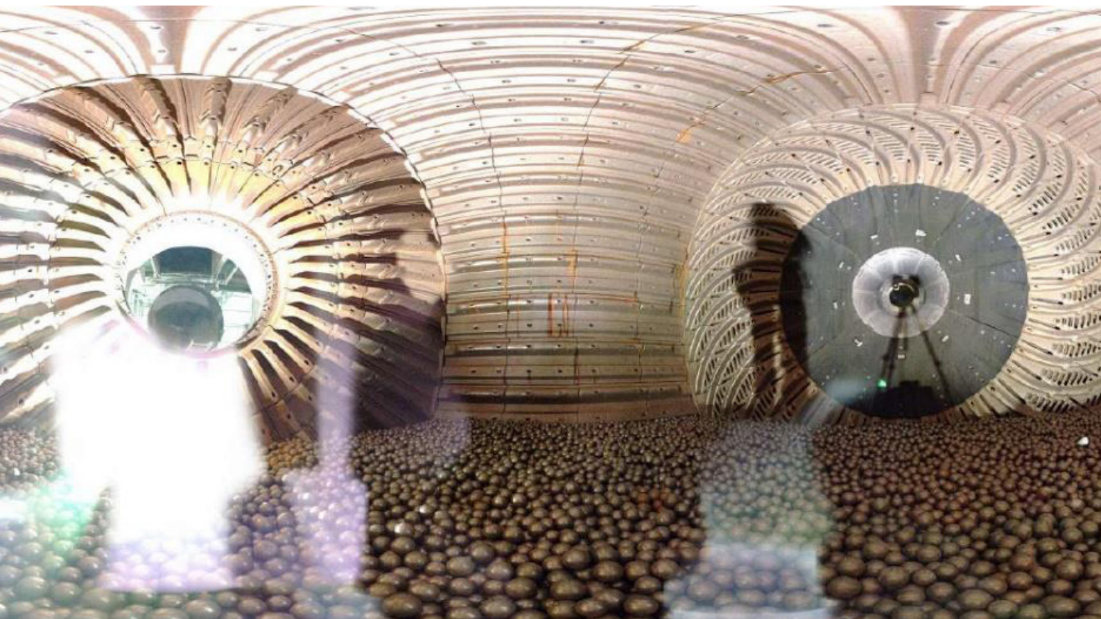
Image 7 – The New Stage 1 Liner Designed Installed in April 2018
