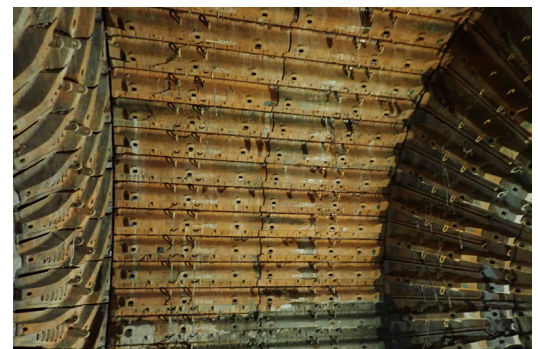
New installation with loose corner liners eliminated
