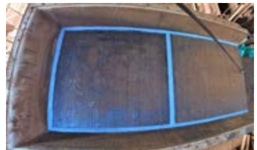
Bradken Duaplate DX 8/8 liner installed
